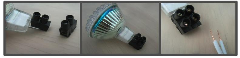
Loosen the screw fastening at the cut side of the terminals, slide them onto the spotlight connections then gently-but-firmly tighten the screws. The opposite screw connector should remain closed until the light is fitted. Once the bulb is fitted open the opposite screws, ready to receive the bared ends of the 2-core wire.
